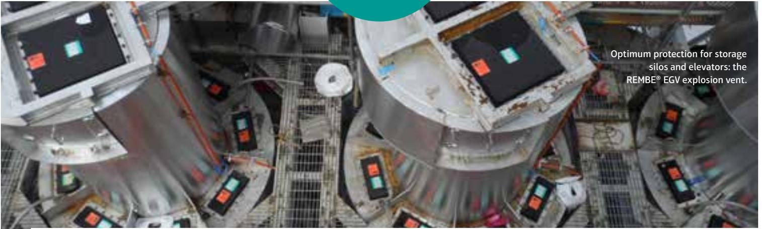
Optimum protection for storage silos and elevators: the REMBE® EGV explosion vent.
