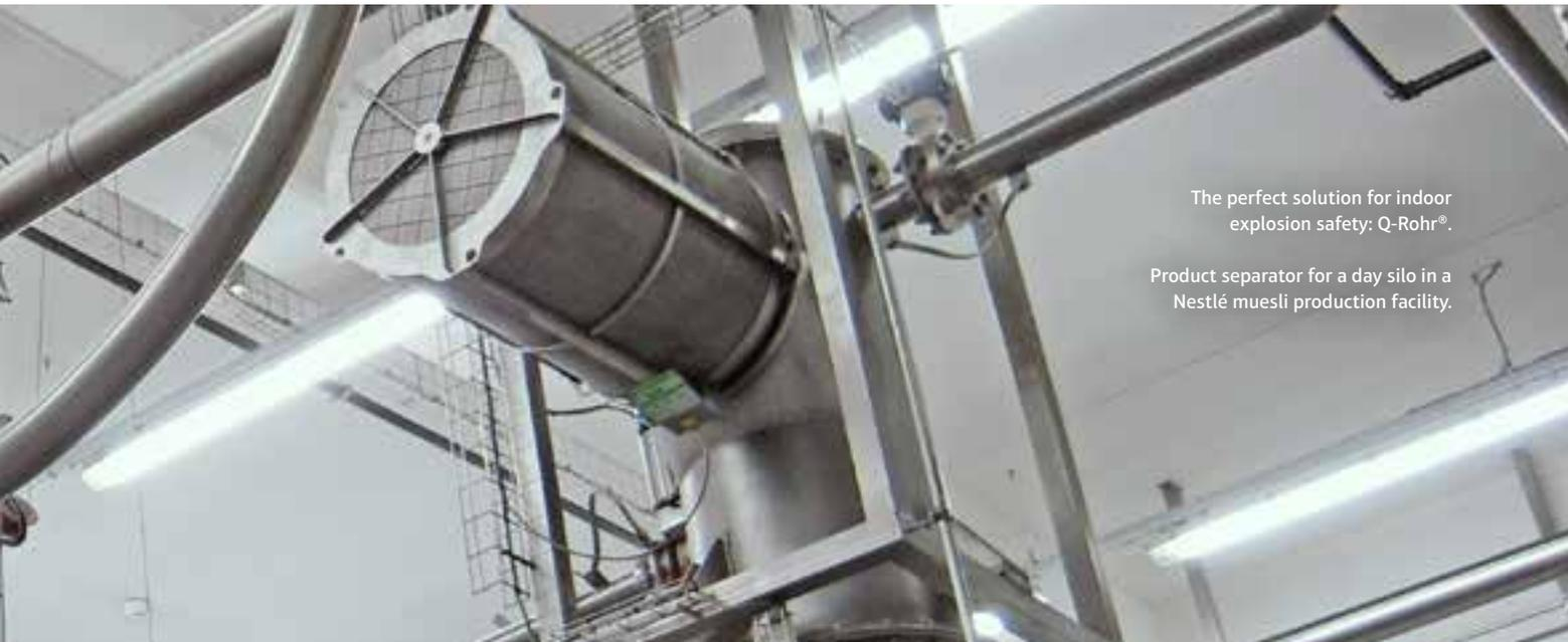
The perfect solution for indoor explosion safety: Q-Rohr®.
